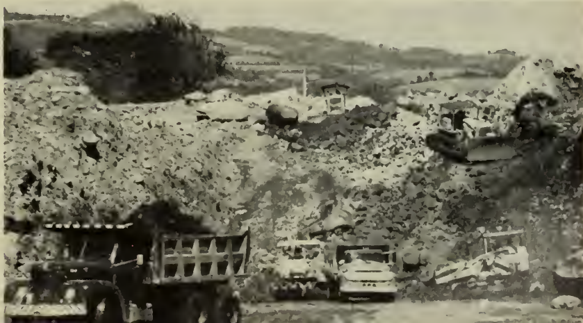
CBs helped clear Rio Reventado Channel in Costa Rica to divert mud-slides.
